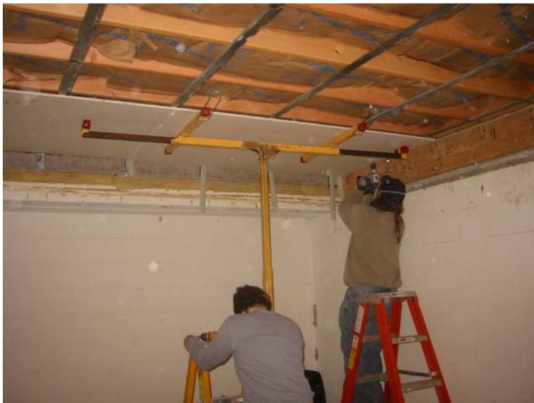
**Figure 4:** Partially installed resilient ceiling
