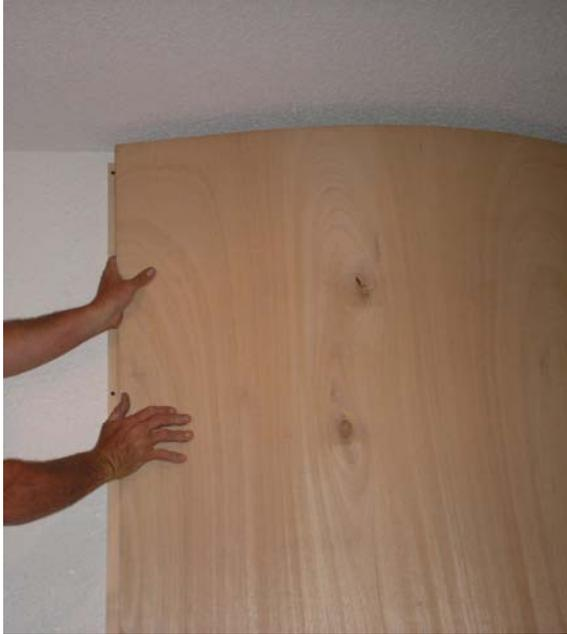
excessive at lower figures, although they lessen as the plywood or Masonite warps to form, and at about 30cm (one foot) the panel starts to become a semi-circle, which yields poorer diffusion, and probably less bass absorption.
