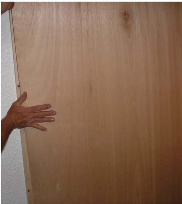
When the sheet is compressed between side boards at 118cm (46-1/2 inches), it takes the shape of an ellipse, reflecting medium to high frequency sound at all possible angles from 0 to 30 degrees, as an ellipse is made up of parts of an infinite number of circles, as with the edge of a football. This works with any width of panel - make the inside of the vertical mounts **3% less** than the width of the panel.
